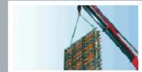
Installation and assembly of wall armoring elements
