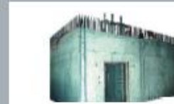
A vault room after filling with concrete mixture and de-panelling
