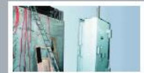
Installation and assembly of vault door
