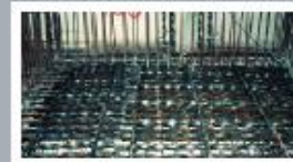
Installation of floor armoring elements
